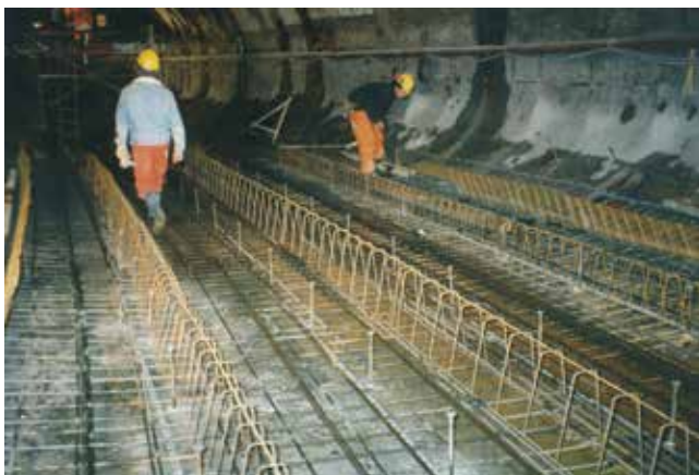
BKW Tunnel BKW tunnel
