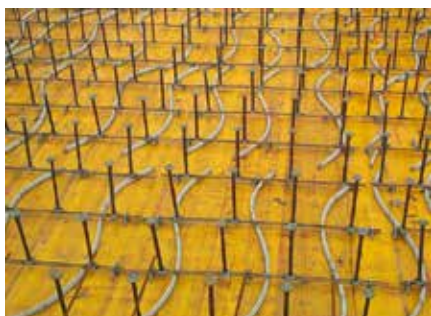
ancoPLUS®-Schubbewehrung / ancoPLUS® - shear reinforcement
