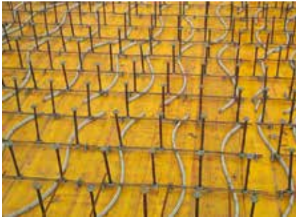
ancoPLUS®-Schubbewehrung / ancoPLUS® - shear reinforcement
