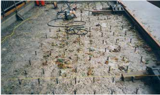
Brückensanierung in Olten Bridge renovation in Olten
