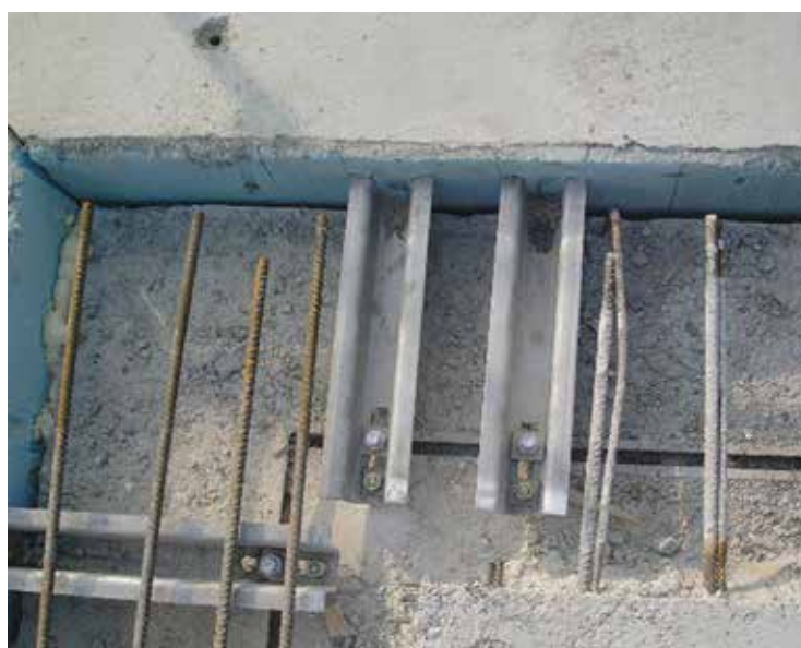
Dachrandelemente - Eckdetail Verankerung. Roof Edge Elements – Anchoring Corner Detail.
