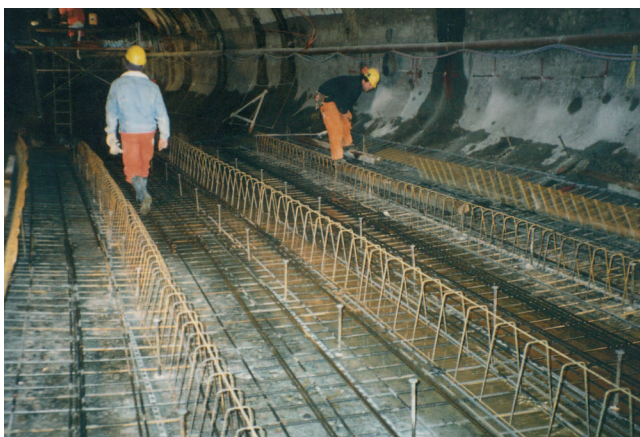
BKW Tunnel BKW tunnel
